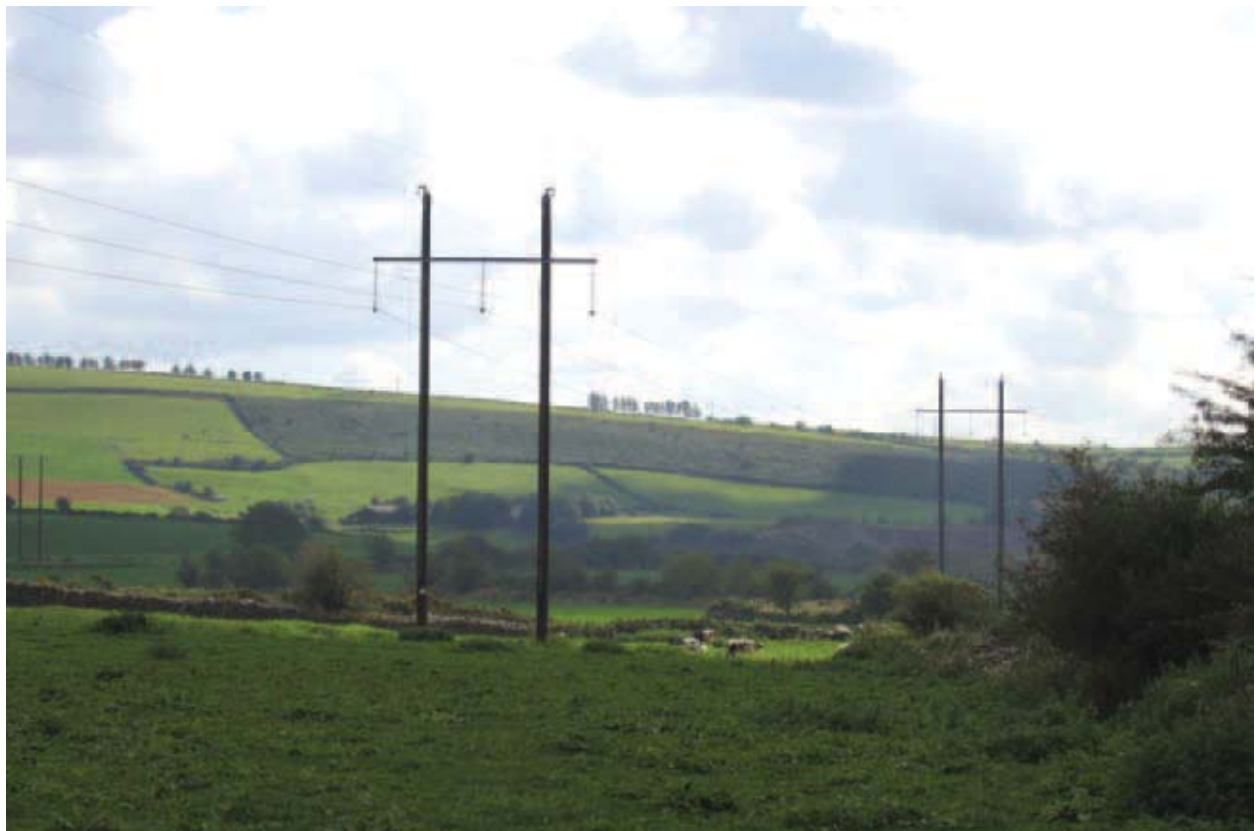
Figure 3.3: An Existing 110kV Single Circuit Line
