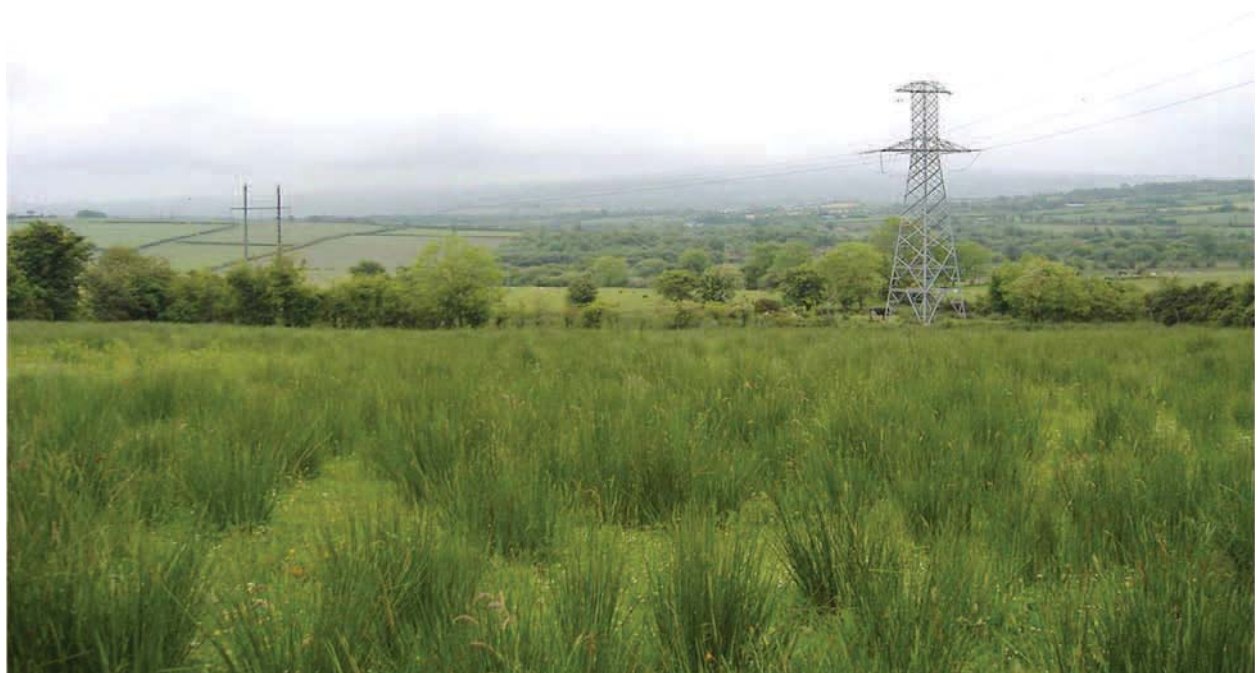
Figure 3.4: A 110kV Line Lattice Steel Angle Tower
