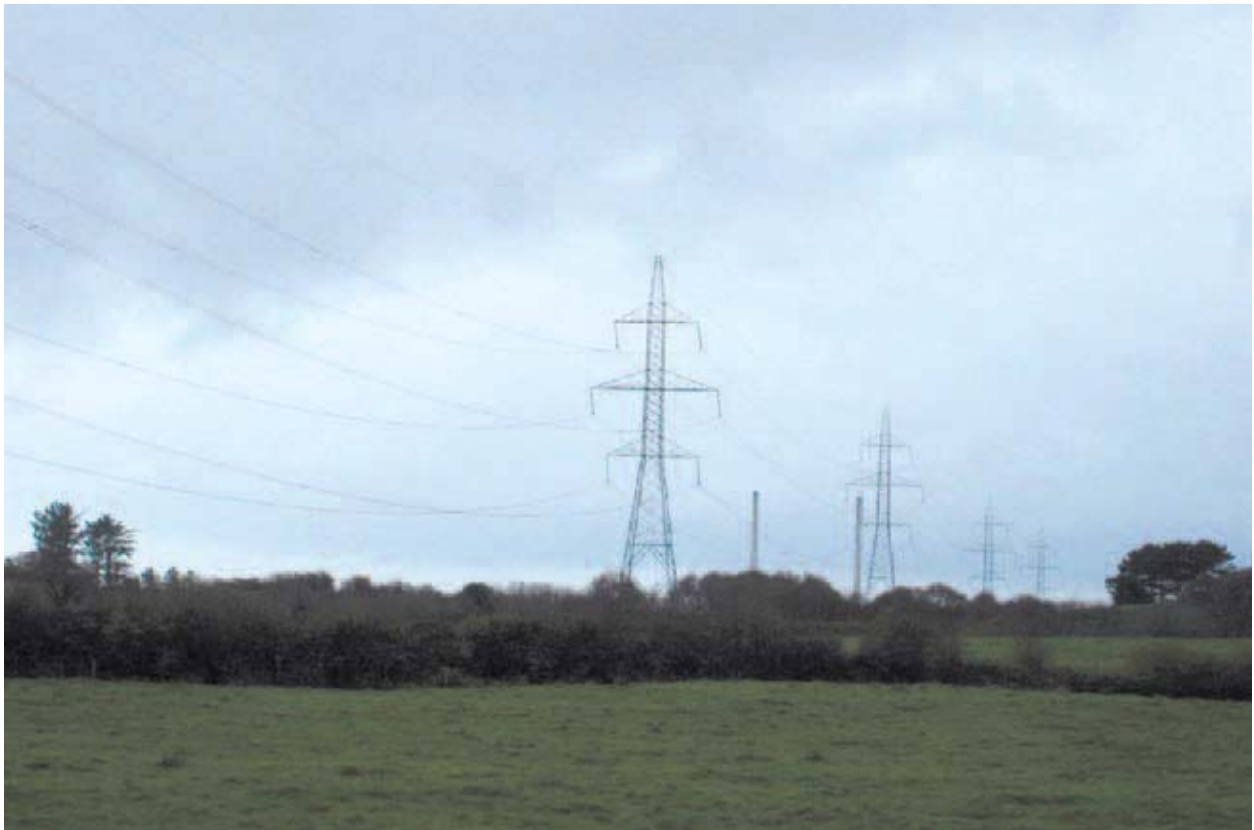
Figure 3.2: Existing 400kV Double Circuit Line (near Moneypoint Generating Station, Co. Clare)
